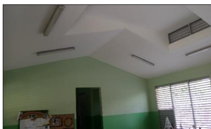
Vista interior inicial
