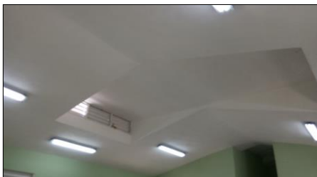
Vista interior inicial
